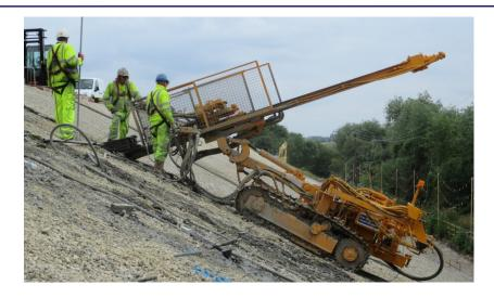
Soil nailing slope stabilisation to support critical embankments that were constructed to new steeper angles on the M1 Managed Motorway contract J39—J42 near Wakefield for Highways England.
